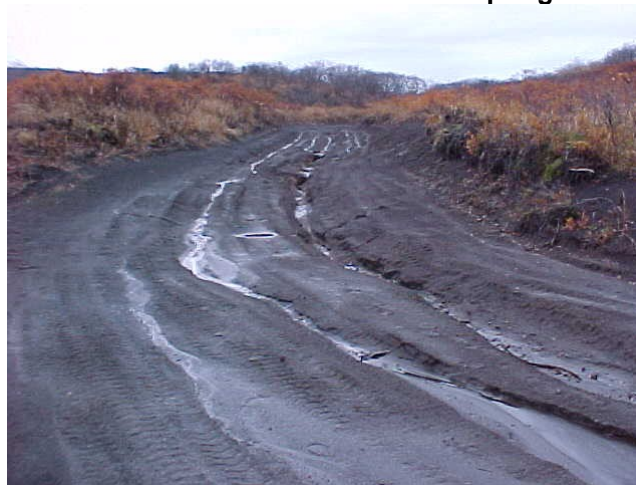
Photo 3: Erosion damage to the road out of Chignik Lake. Photo taken on November 5, 2002.
